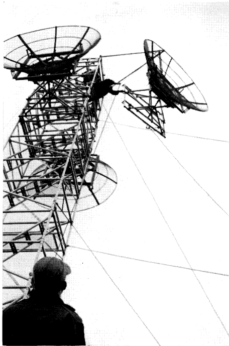
A temporary transmission path testing tower was the first big structure put up at each White Alice site.
