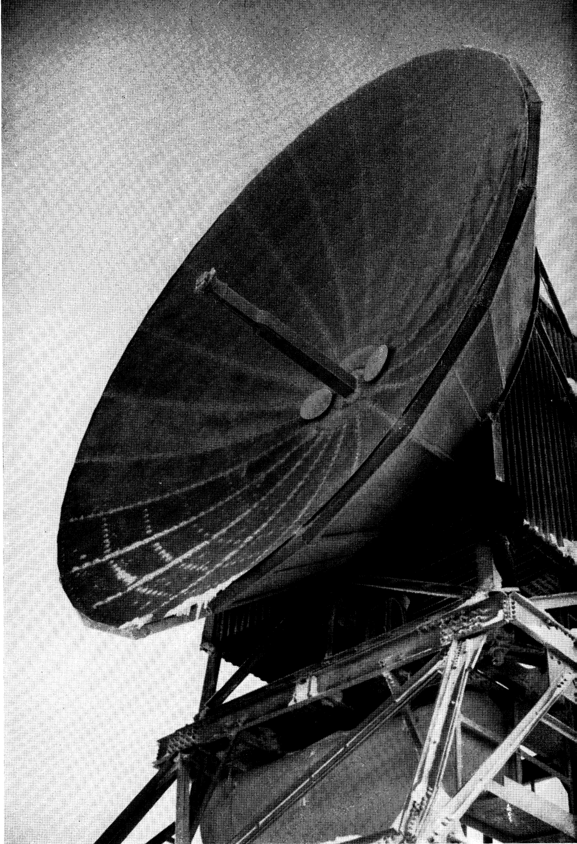
A "dish" antenna, one of the two types used in the White Alice beyond horizon system. Its face measures 30 feet across.
