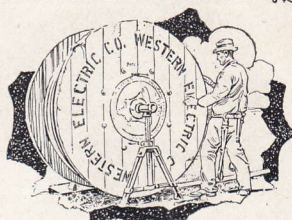
Paying Out Aerial Cable
