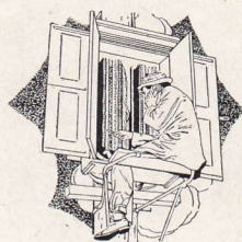
Lineman at Terminal Box
