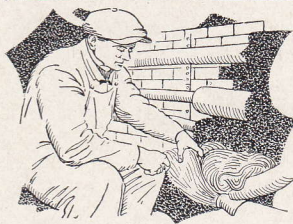
Splicing Underground Cable
