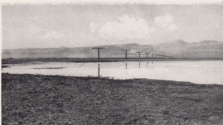
Transcontinental Telephone Line Crossing Humboldt Flats, Nev.
