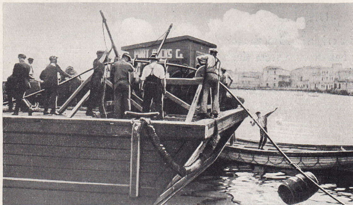
Laying One of the Shore-ends of the Havana-Key West Cable in Havana Harbor
