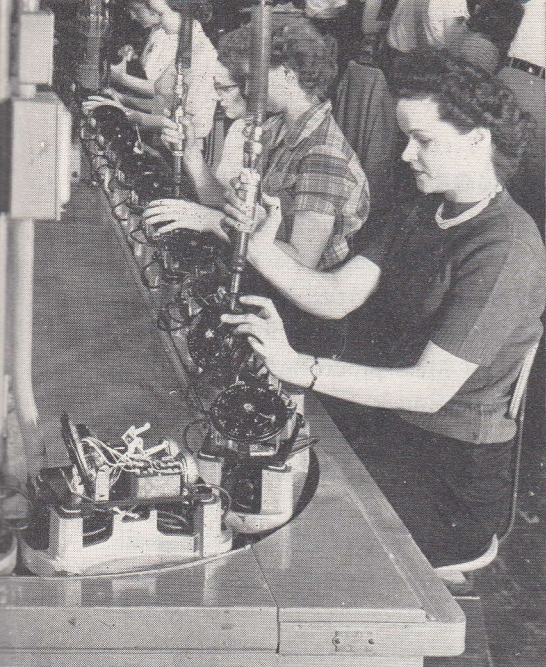
Manufacture of the familiar Bell telephone instrument is centered in the modern Western Electric plant located in Indianapolis. These girls are performing one of the many assembly operations that are required.
