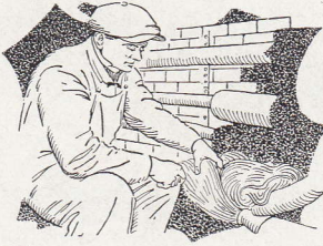
Splicing Underground Cable
