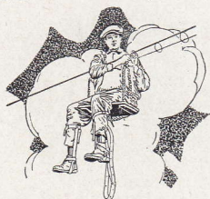
Twisting Rings on Messenger Strand
