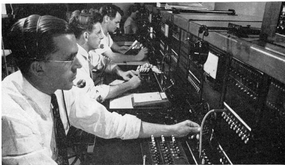
Technicians check for trouble at a test desk in a central office. Preventive maintenance, outside as well as inside telephone offices, helps provide good service.
