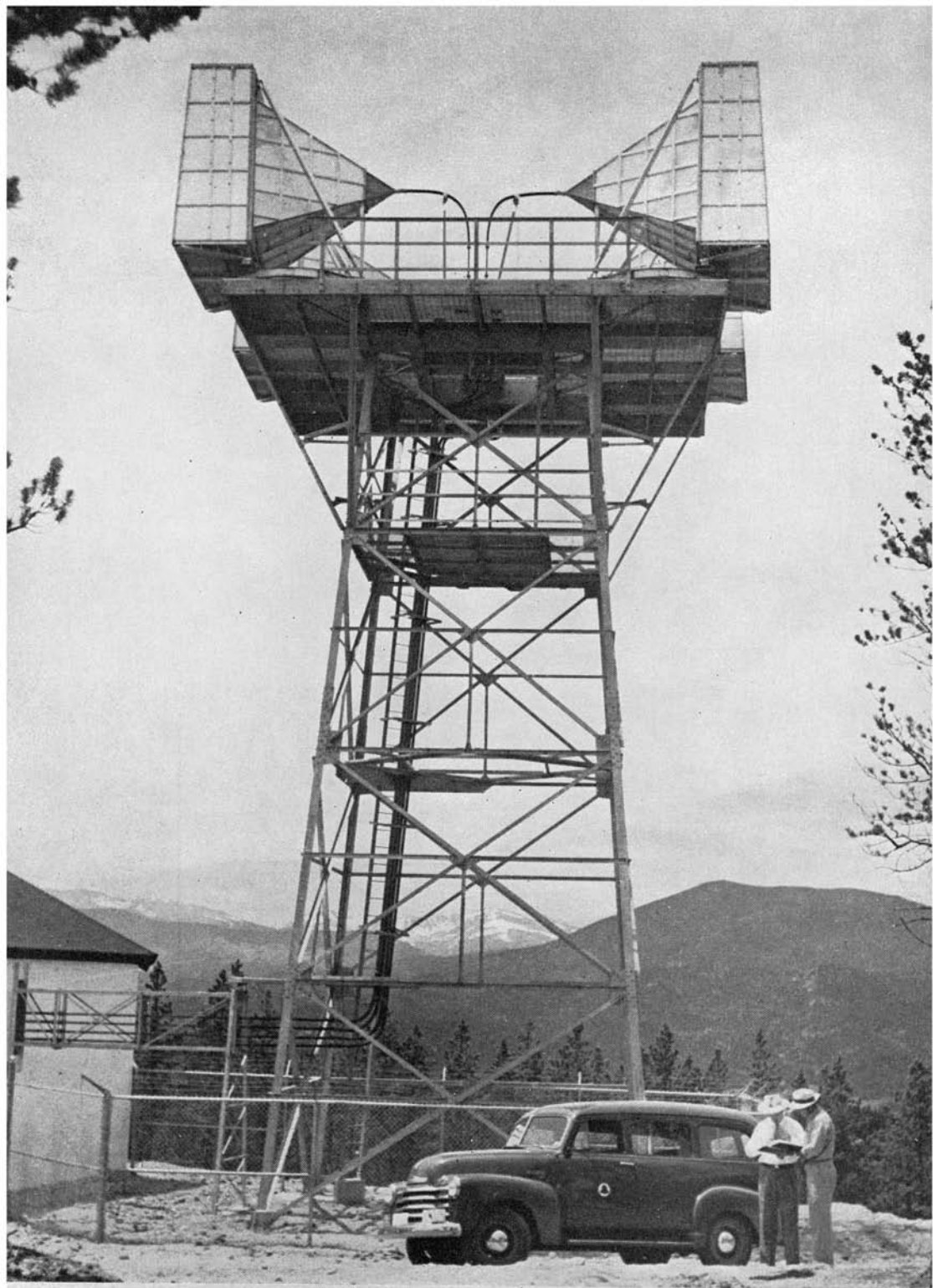
This radio-relay station on Buckhorn Mountain in Colorado is one of 107 in the Bell System's transcontinental microwave system. Flashed from station to station, telephone calls and television programs first spanned the continent by air in 1951.
