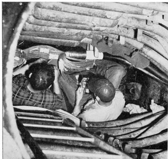
Left, splicers "cutting in" wires in a new cable, below the street in manhole. Right, Bell telephone installer connects drop wire to new subscriber's home.
