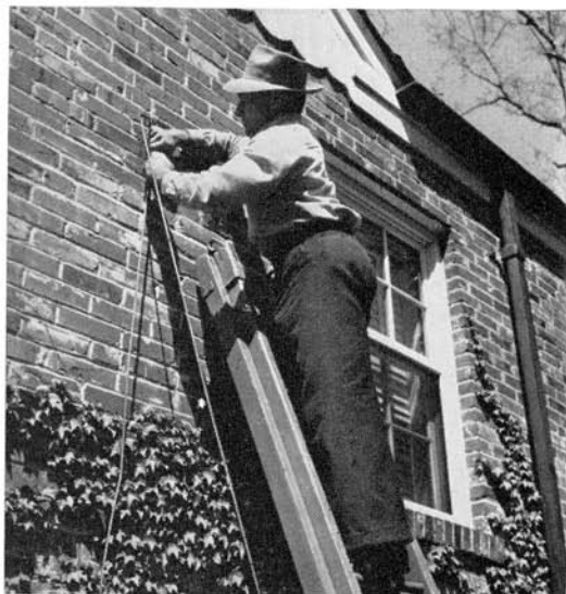
Left, splicers "cutting in" wires in a new cable, below the street in manhole. Right, Bell telephone installer connects drop wire to new subscriber's home.
