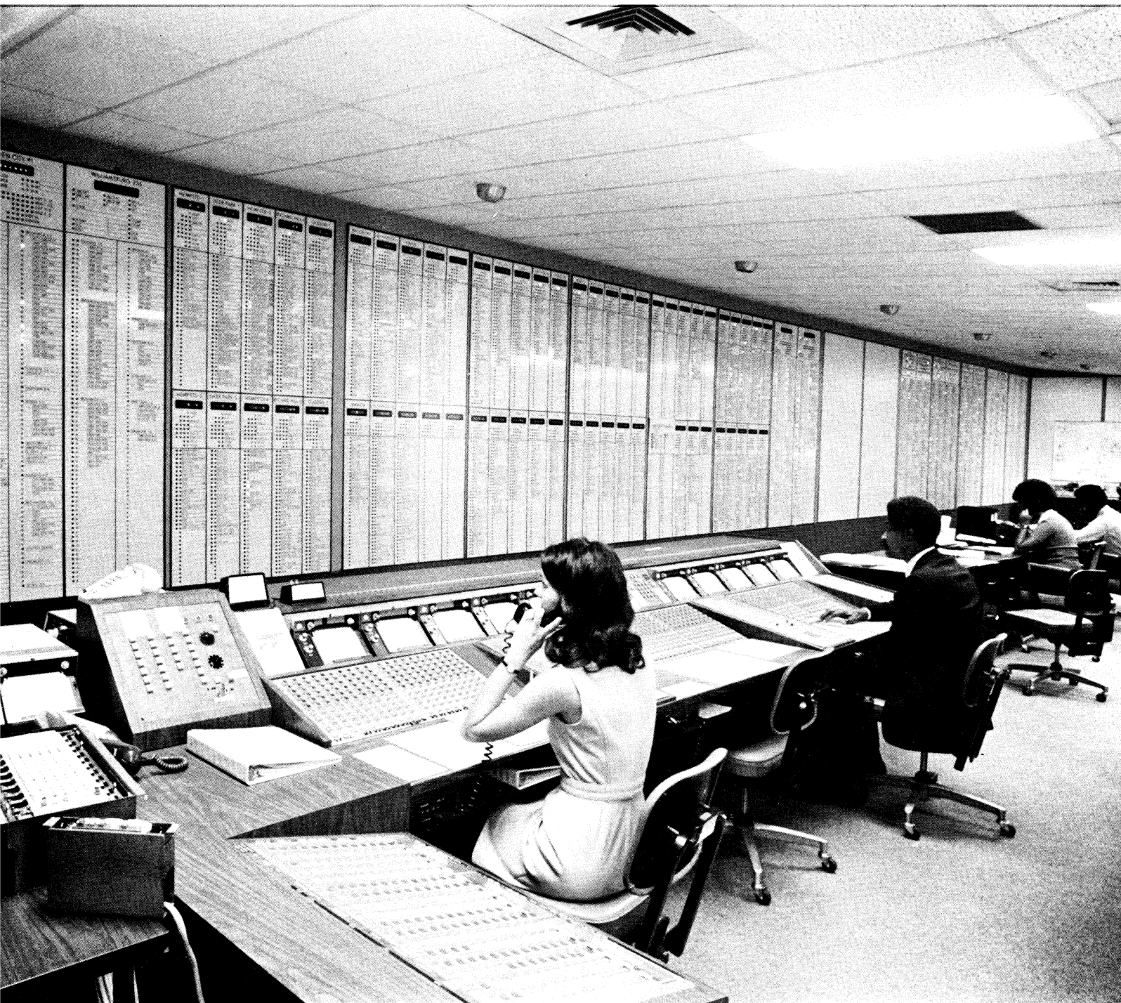
At the Network Management Center on East 38th Street, New York City, consoles and display boards help personnel monitor and control the operation of the downstate New York network. The Center is jointly operated by New York Telephone and AT&T Long Lines.
