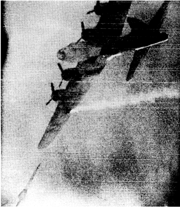
A Nike Ajax missile approaching (from the left) and destroying a drone B17 bomber (at right) in tests at the White Sands Missile Range, New Mexico, in 1952.
