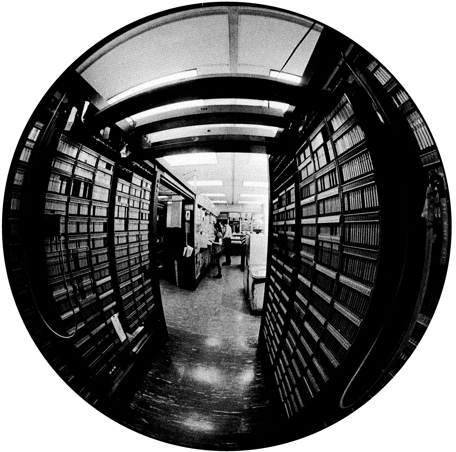
The electronic switching systems of the 1960s exploited the data processing technique of programming to offer unprecedented speed and reliability, and a host of new services that can be added by modifying the program. This fisheye-lens photo shows frames in a typical No. 1 ESS office.
